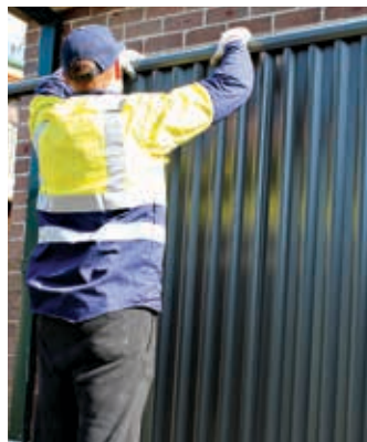
Position 4th sheet. Gentle force can be used.
