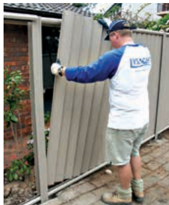
Position 3rd sheet. Gentle force can be used.
