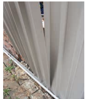
Place 2nd sheet into bottom rail, ensuring there is sufficient overlap.
