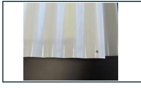
13 Fix the Fibreglass diffuser along its length using the Stormtite screws. Repeat for all remaining skylights.
