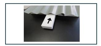
14 Once all cavities have been filled with EPS insulation blocks, cut the Z Flashing for the gutter end to the correct length and install it as normal by fixing to the roof panels using rivets from the underside and through the valleys at the top at 300mm centres. Do not rivet the overlap section as you will need this to lift to insert the foam infill in the next step
