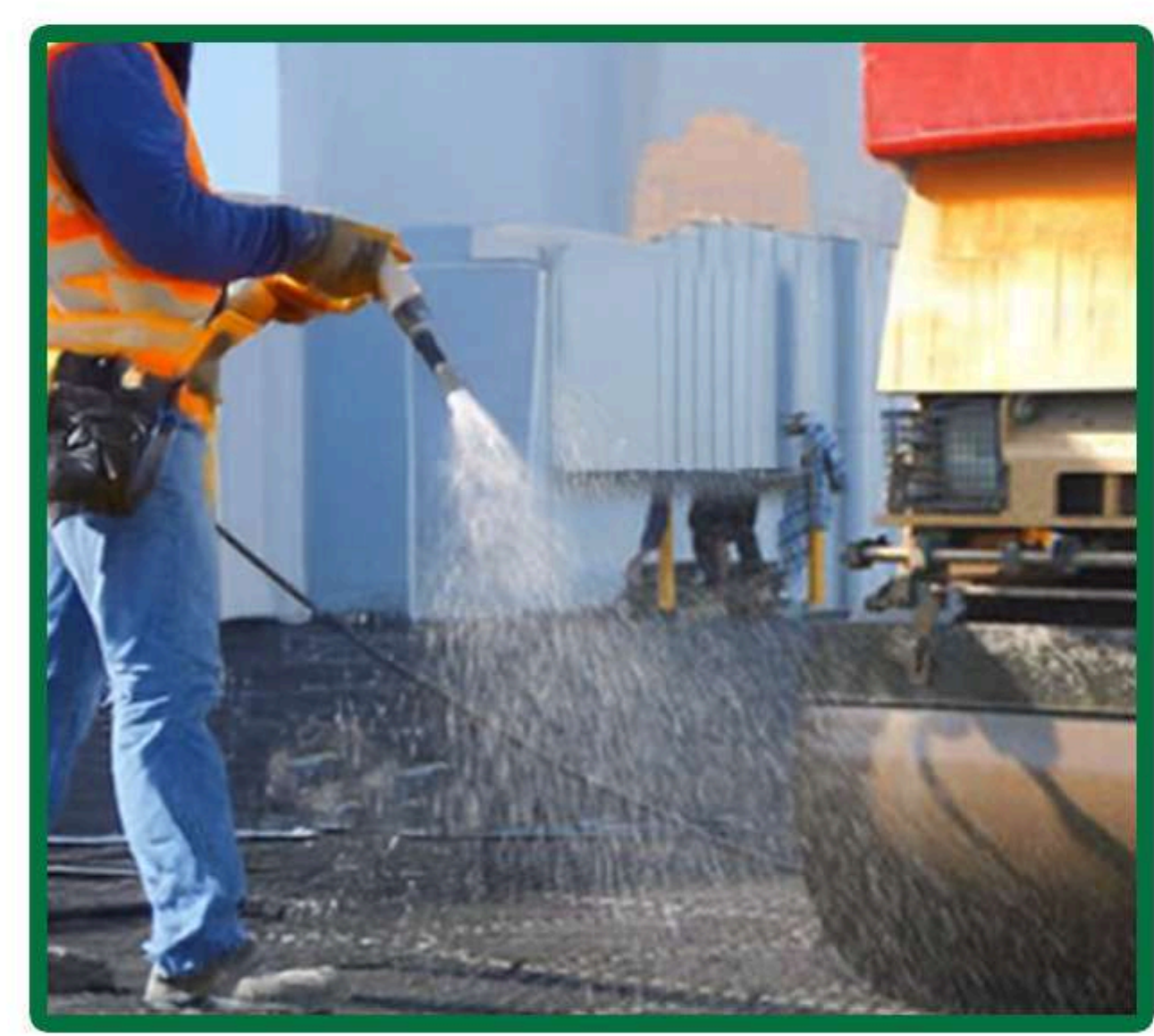
Figure 11 - Rolling in TREXLOK grid before concrete fill.
