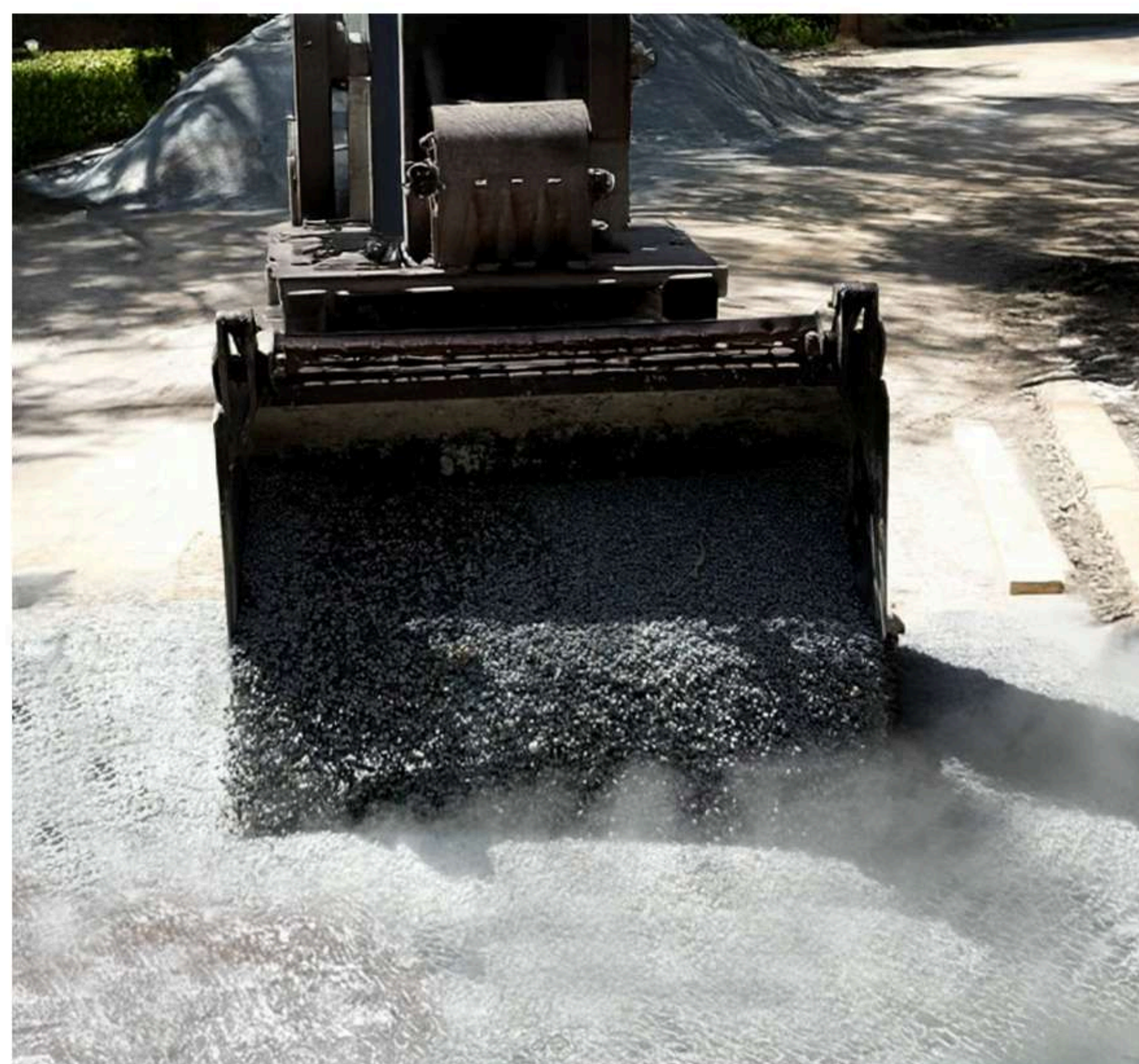
Figure 27 - Filling TREX with aggregate.
