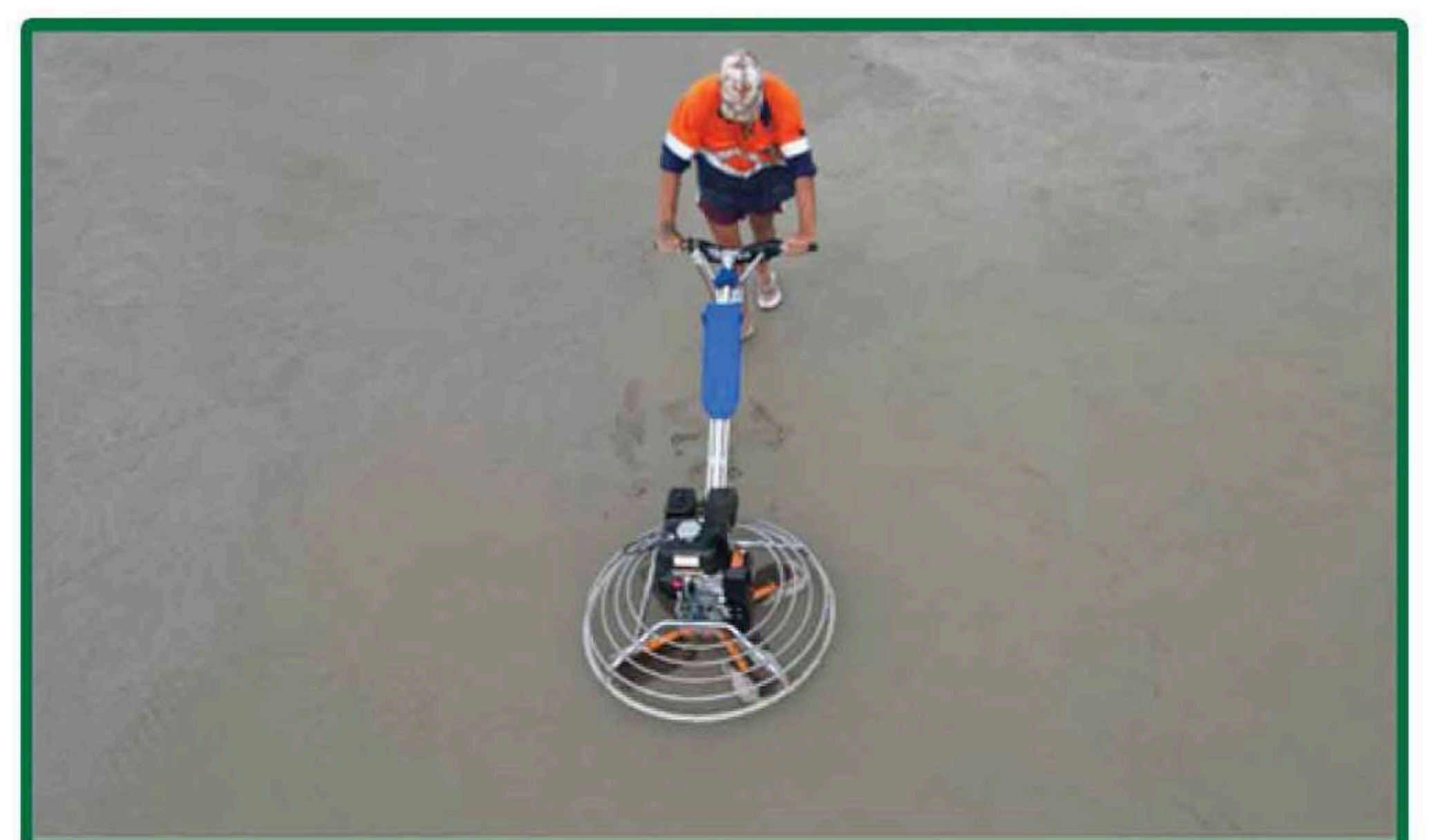
Figure 15 - Concrete finishing work in sections, using a trowel machine.
