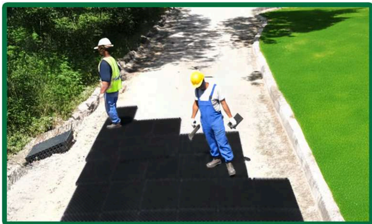
Figure 23 - laying TREX pattern.
