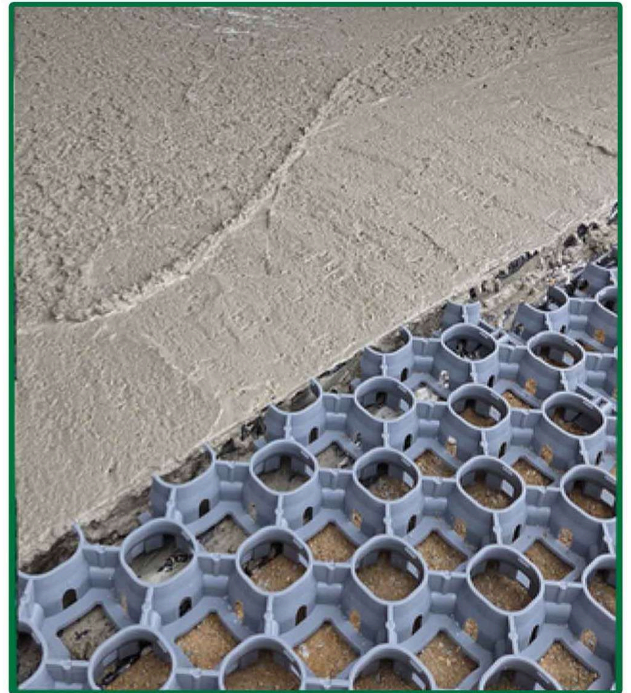
Figure 12 - Concrete mix should be approx 120 slump 10mm stone for easy pouring into TREXLOK.
