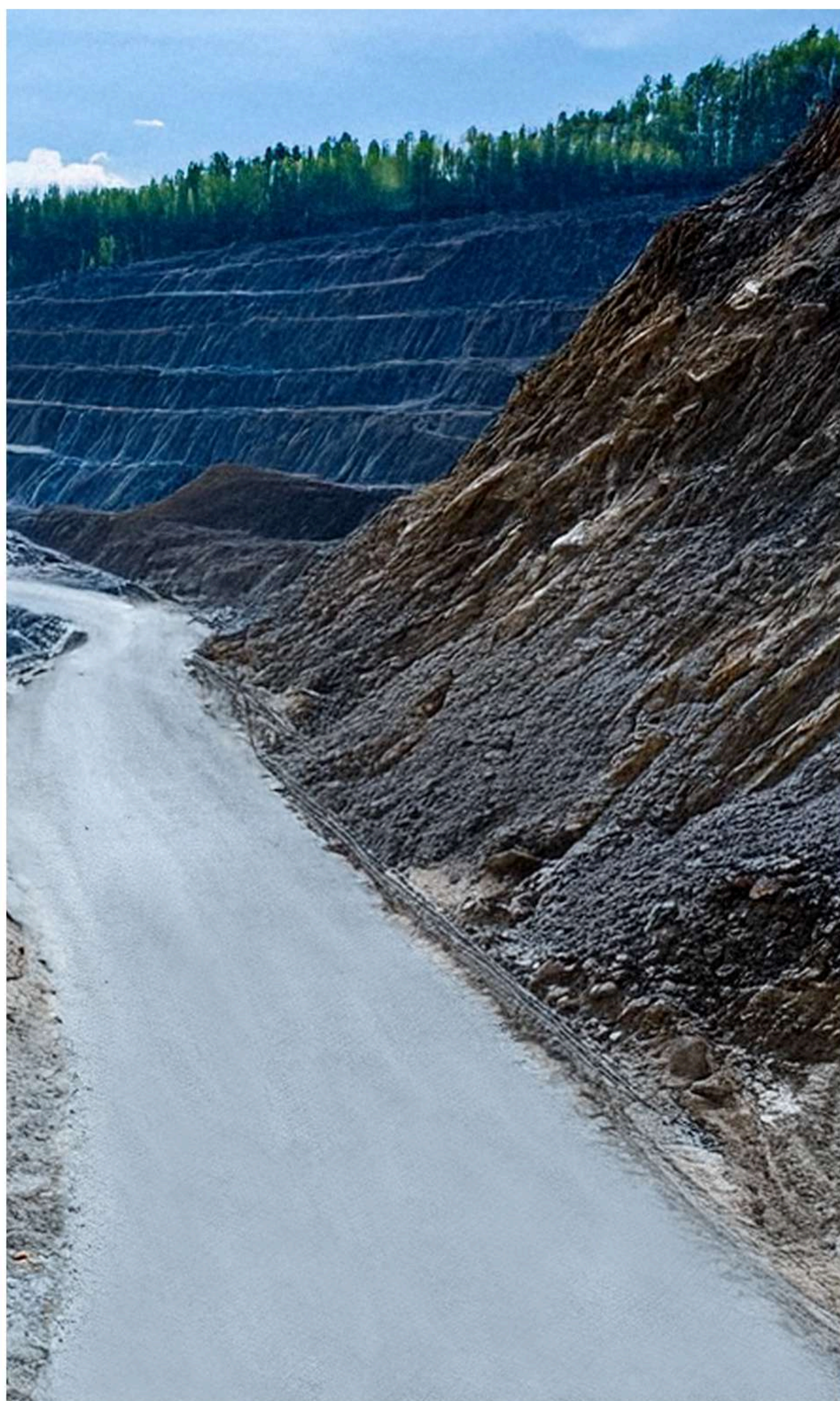
Figure 30 - Completed TREX permeable unbound pavement.
