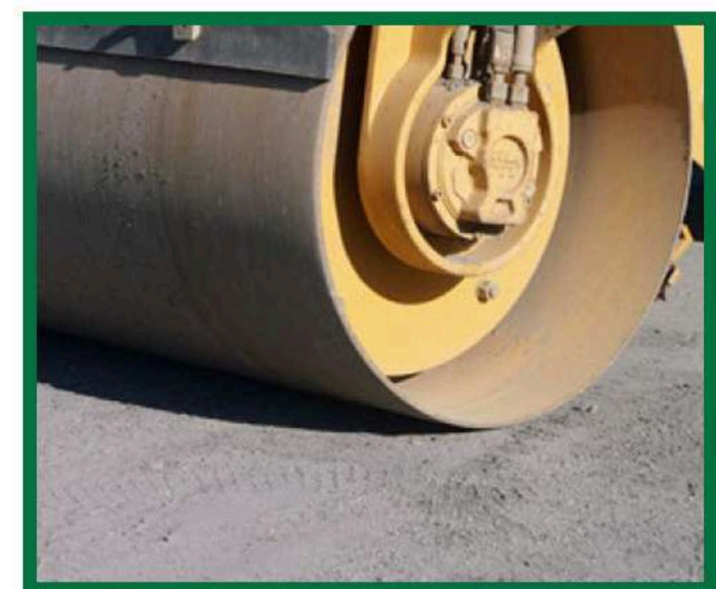
Figure 4 - Subbase Preparation: Spreading and leveling road base prior to compaction. Compacted and watered, ready for TREXLOK installation
