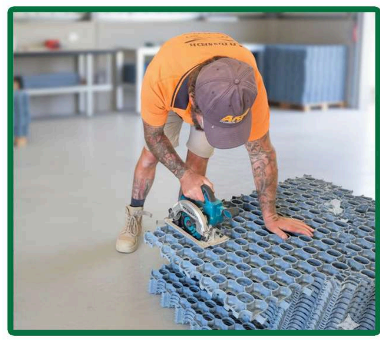
Figure 10 - Cutting TREXLOK to fit around objects easily cut with a circular saw or grinder.
