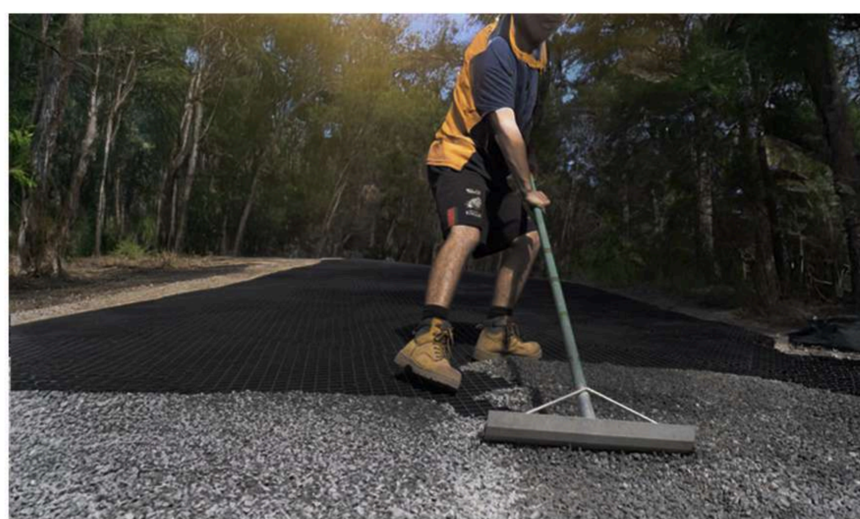
Figure 29 - Use a concrete rake to help spread evenly.
