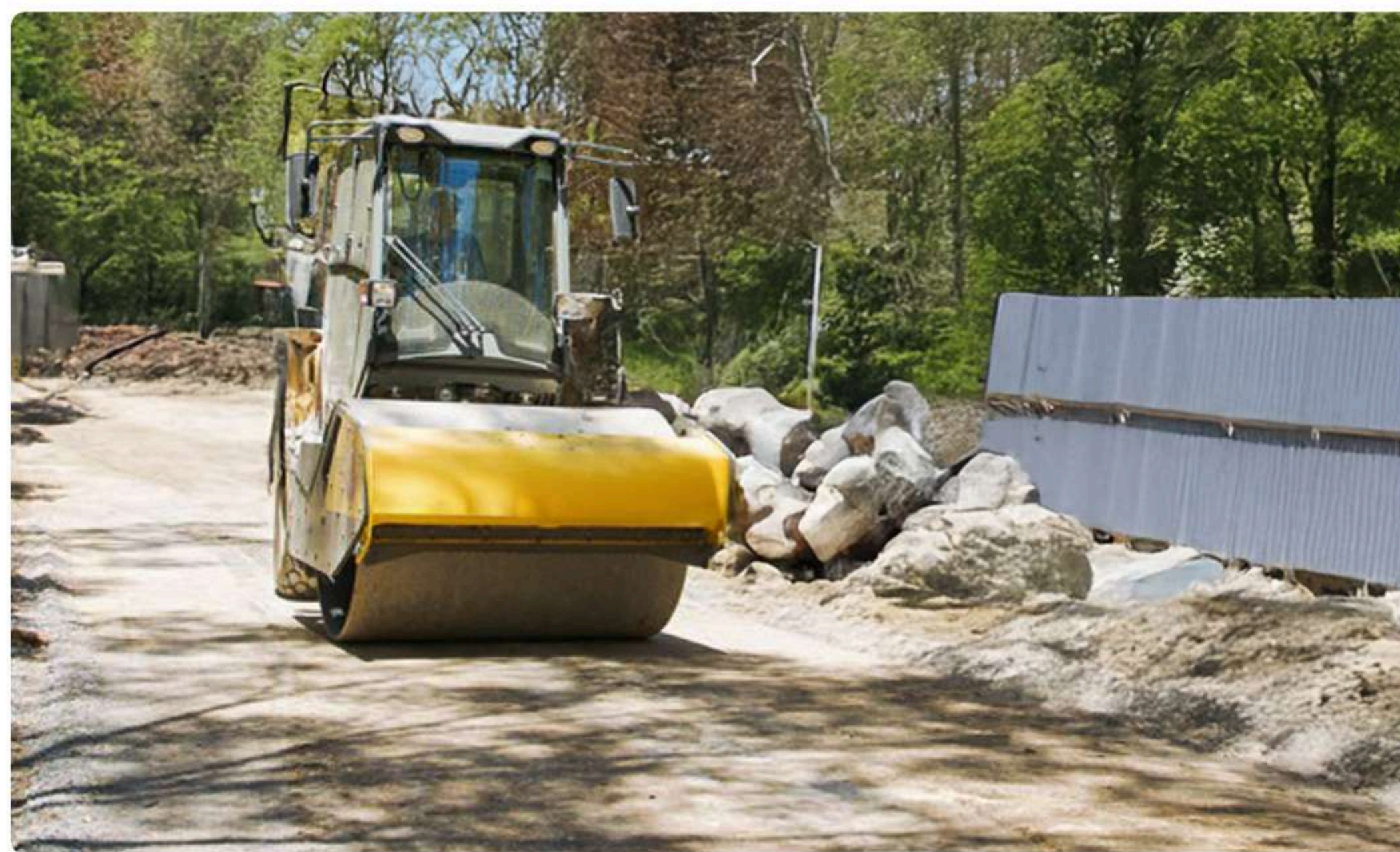
Figure 16 - Subgrade Preparation: Graded and compacted.
