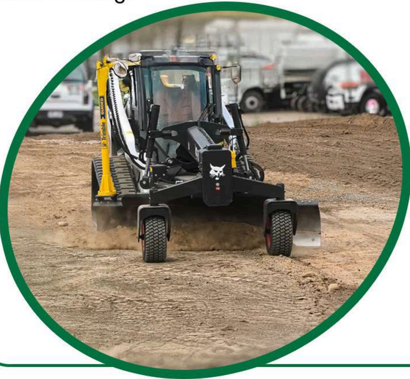
Figure 1 - Subgrade Preparation: Graded Prior to compaction and levelling.
