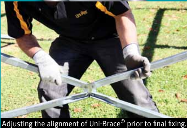
Screwing diagonals together.
