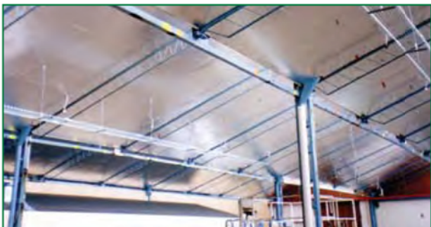
KOOKABURRA MANUFACTURING PLANT- REFURBISHMENT Here FOILBOARD® INSULATION PANEL was used to drastically improve the thermal efficiency of this factory. The pure aluminium foil laminated to FOILBOARD® also helped increase the ambient light whilst adding to the aesthetics.
