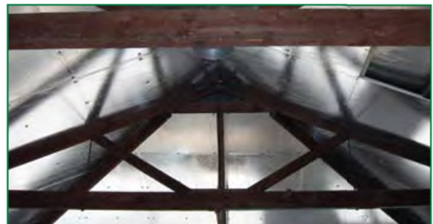
B.P.S. Technical Bookshop FOILBOARD® INSULATION PANEL was used here to retro fit an old storehouse to a retail outlet. The developers were keen to maintain the industrial look of the building whilst drastically improving thermal efficiency.
